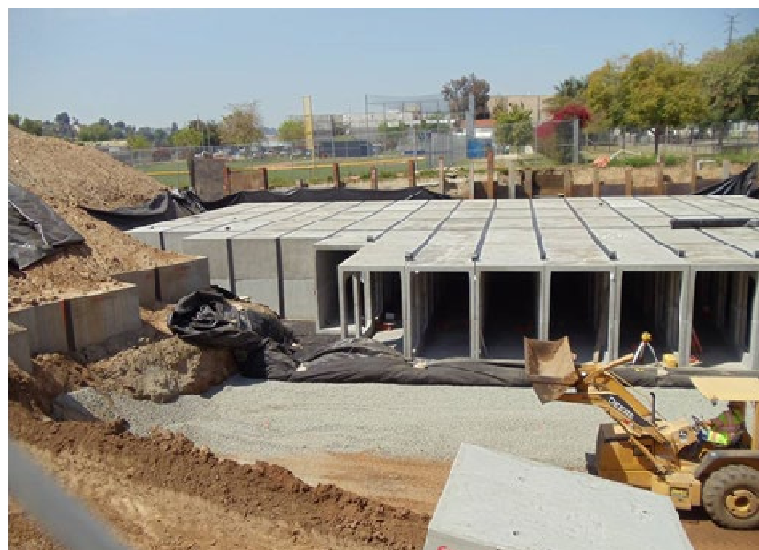
Figure 1. Subsurface design of an infiltration basin, mid-construction.
