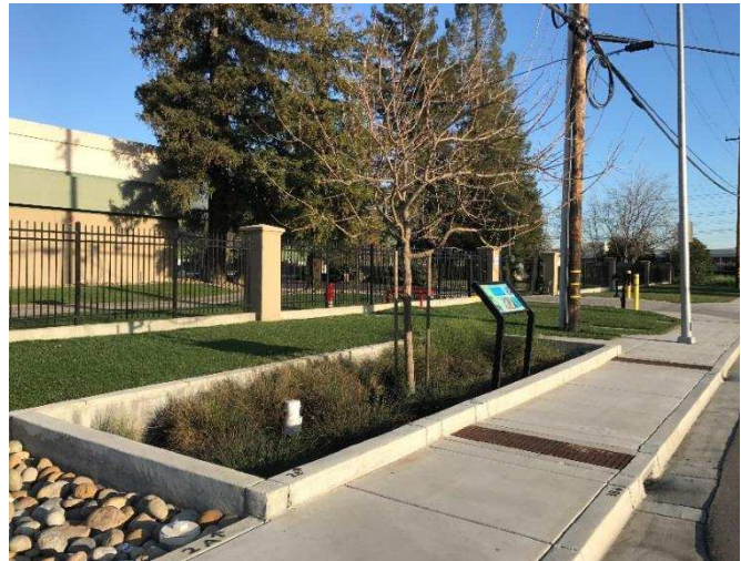
Source: City of Fremont Figure 1. Tree-well filter designed by the City of Fremont
