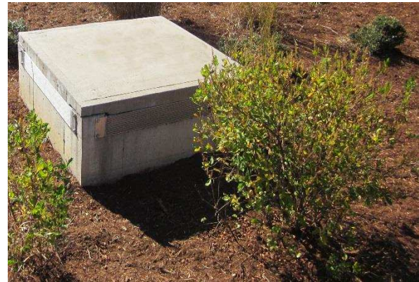
Figure 5. Example of an outlet with 5 mm screen.
