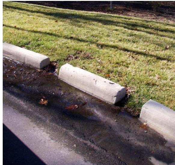
Figure 4. Example of filter strip as pretreatment
