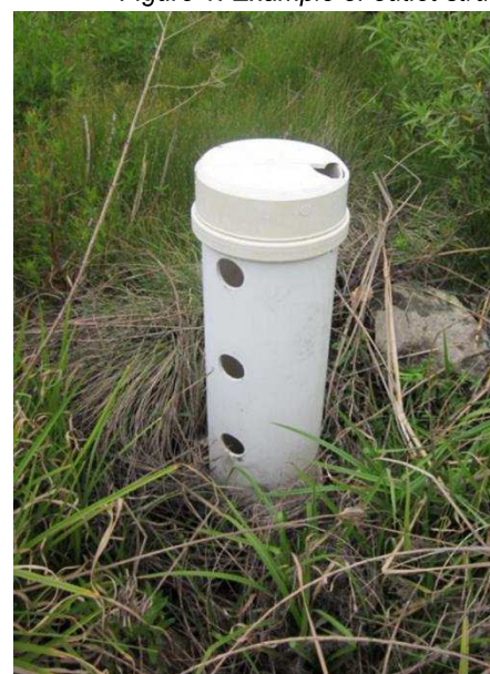
Figure 2. Variable flow outlet structure.
