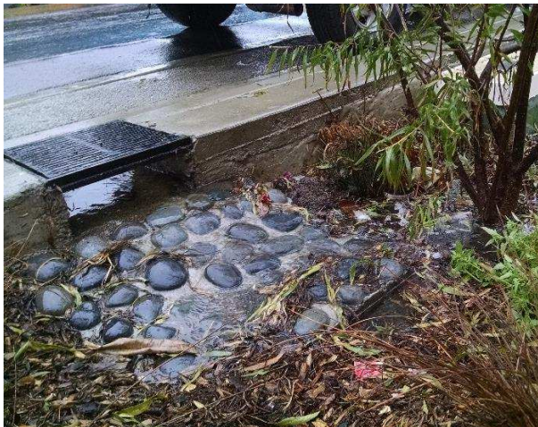
Figure 9. Example of mortared cobble for pretreatment in a bioretention inlet with a curb cut.
