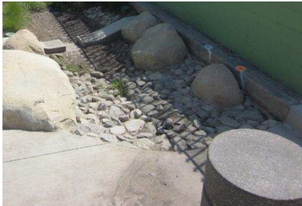
Figure 3. Example of a forebay as pretreatment
