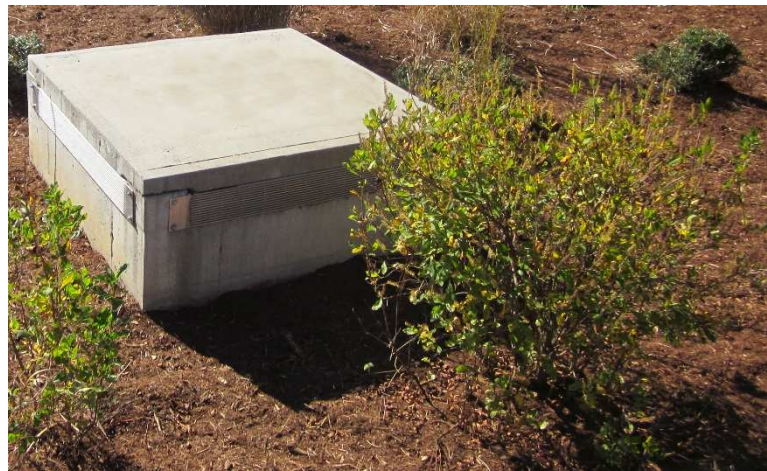
Figure 3. Example of an outlet with 5 mm screen.
