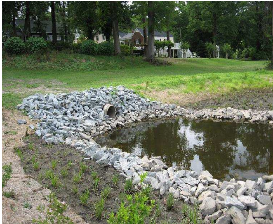
Figure 1. Example forebay. Also note other components of the pond: earthen berm and native vegetation
