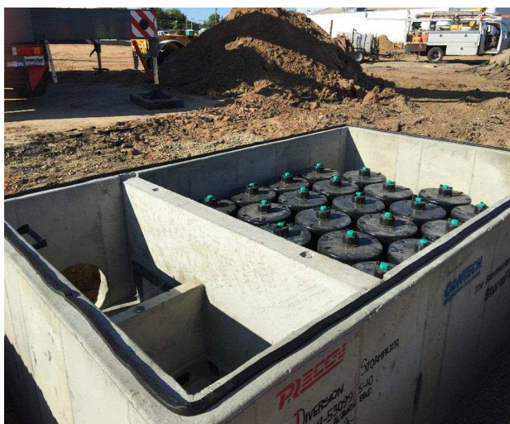
Figure 1. Stormwater media filter vault, mid-construction.
