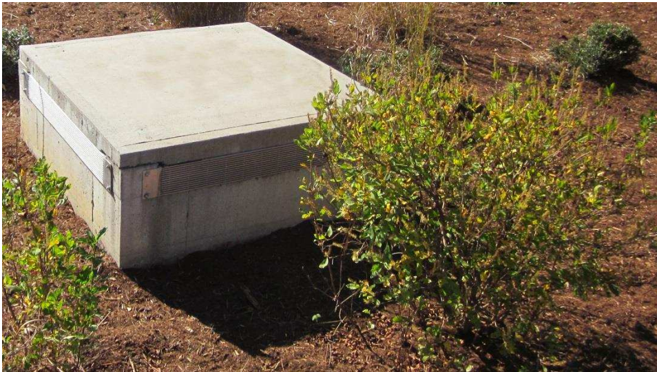
Figure 5. Outlet structure with a 5mm screen.
