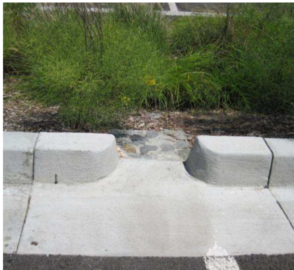
Figure 5. Example of an open curb cut.
