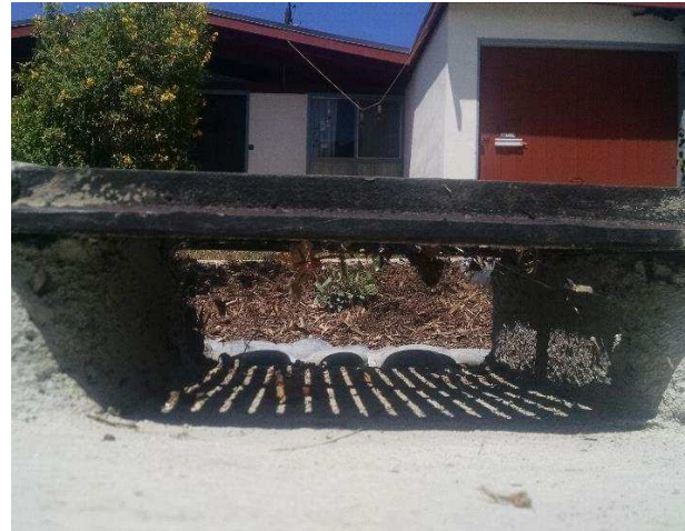
Figure 9. Example of mortared cobble for pretreatment in a bioretention inlet with a curb cut.
